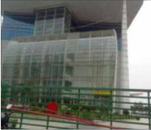
Front view of Building
