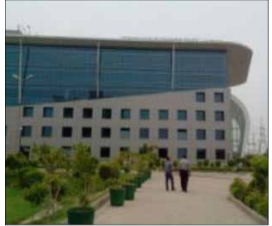
Side view of Building
